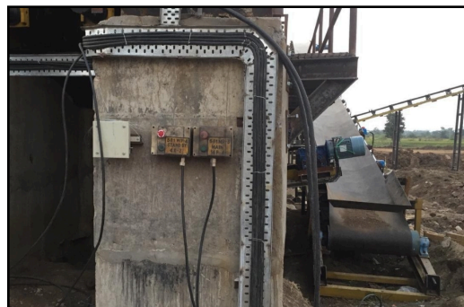
Emergency Stops, Aluminium Armoured Cabling, along with Fully Automatic Control Panel
